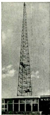
WXEL-TV Cleveland, Ohio. Truscon Self-Supporting Tower, 437 feet high.
